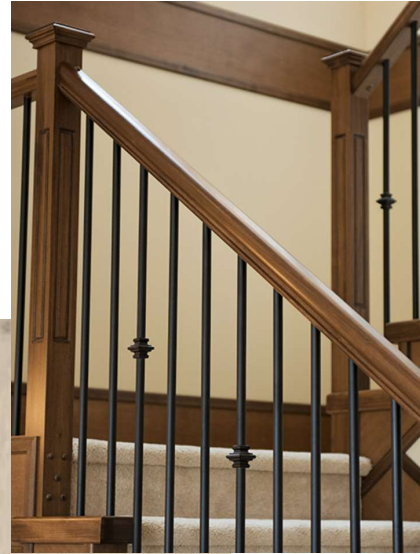
Craftsman handrail and newel post stained to match wood floor, iron pickets
